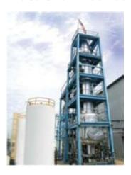
Fractional distillation is used to separate mixtures of miscible liquids, such as ethanol and water. The technical aspects of the fractional distillation process allow mixtures to be returned to their original states with a 99.9% degree of purity.
