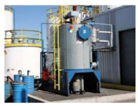
Tradebe's second distillation option is a Solvent Recovery Distillation Unit. This unit has a wiper blade and can handle high solid (<20%) viscous feedstock. This technology can reclaim approximately 40,000 gallons of solvent per month. The Solvent Recovery Distillation Unit is used for smaller batches of solvents received by Tradebe to remove solids and color from the solvent.
